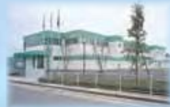
Mie Plant (TA & IT Plant)
